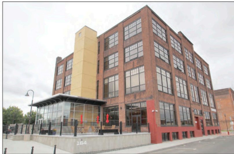
Cubit Building, home to the HCC MGM Culinary Arts Institute, where HCC will be running a cannabis culinary assistant training program April 19 to May 10.
