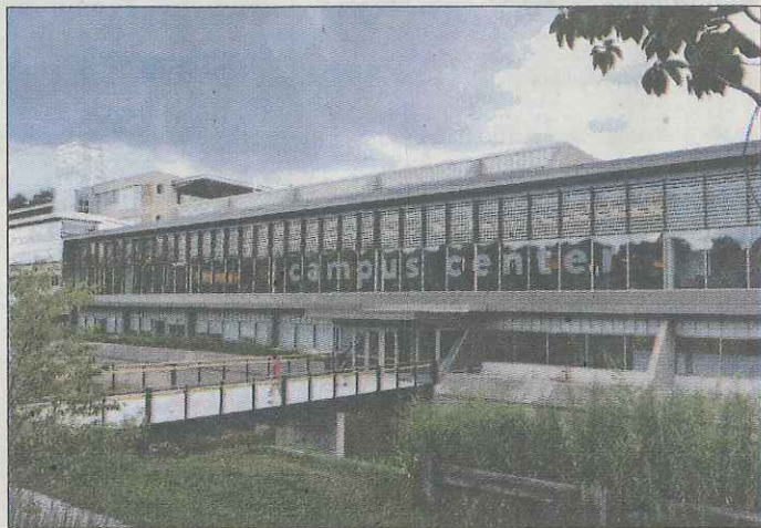
Holyoke Community College's Campus Center.
