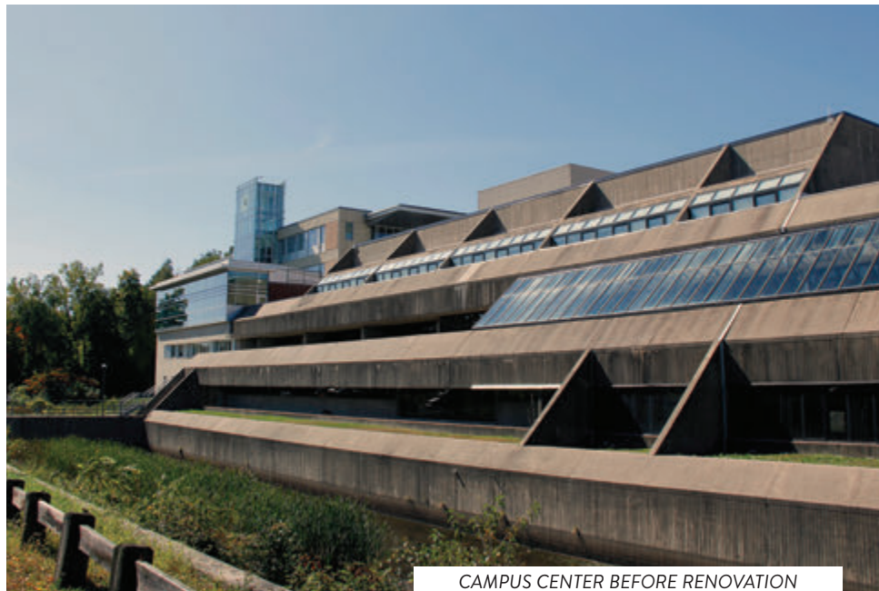
CAMPUS CENTER BEFORE RENOVATION
