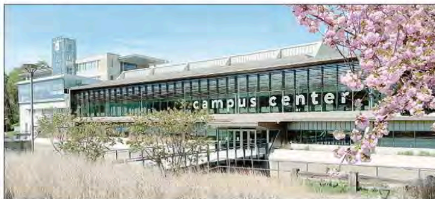
The Holyoke Community College campus offices and fitness center are reopening, though masks will be required for now.
